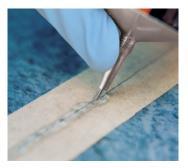
After about 10 minutes the cold-welding liquid on the masking tape is dry and the tape has to be removed steadily backwards at an angle. Swellings in the seam area of the PVC-floor covering will decrease. The result is a barely perceivable seam with a high seam tensile strength. The seam can be walked on after about 30 minutes.
